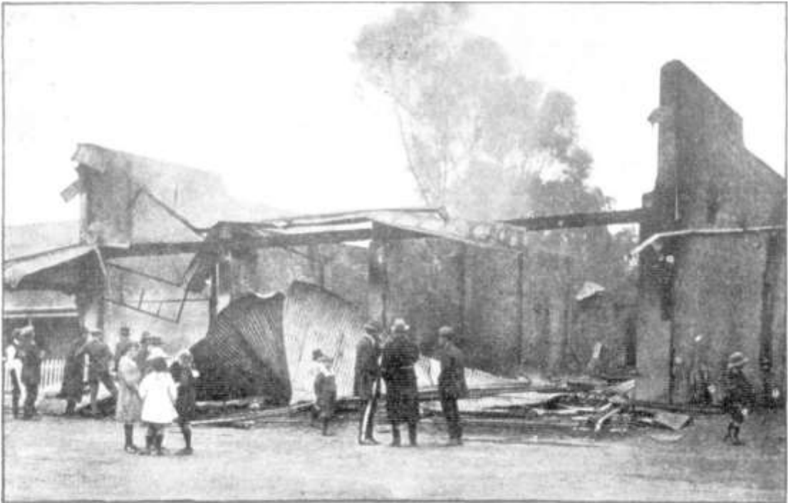
PREMISES OF MESSRS. W. P. MARSHALL & WILLIS BROS. DESTROYED BY FIRE ON MAY 12. Wooler, photo.
